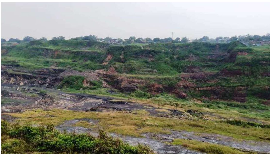
Figure 19: Subsidence area in Bagdigi Mines
